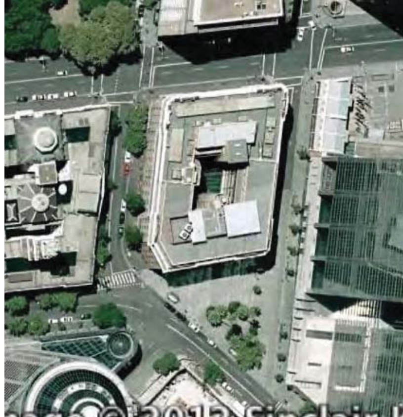
Existing condition: Farrer Place and surrounds
